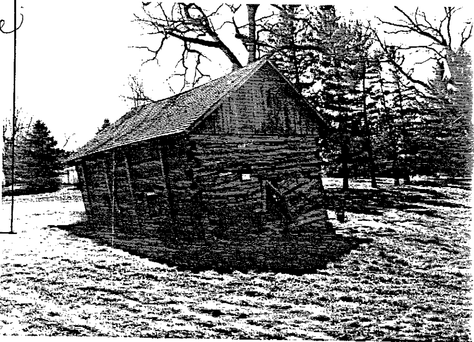
Looking South West (Back side) 251
